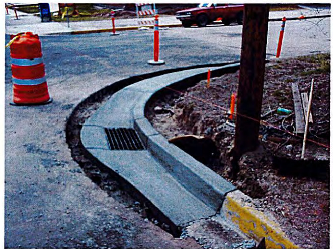
April 10, 2002 New curb & gutter on Center Street.
