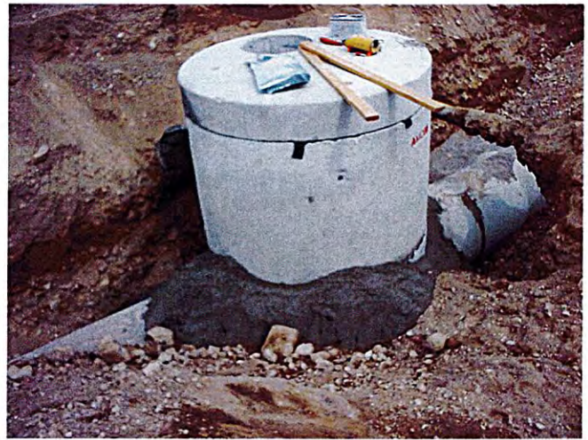
April 8, 2002 Installation of manhole on Center Street.
