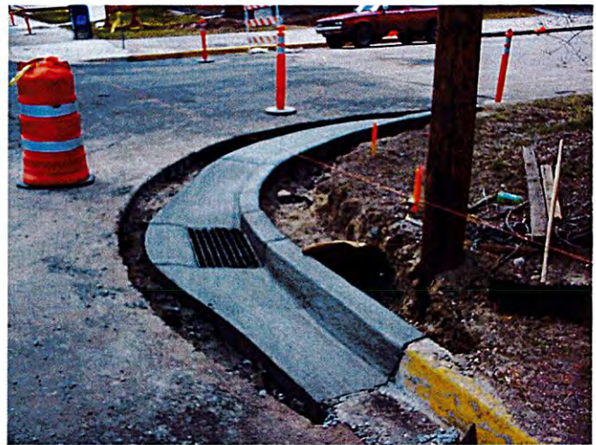
April 10, 2002 New curb & gutter on Center Street.
