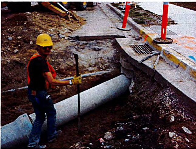
April 8, 2002 Catch basin lateral installation.
