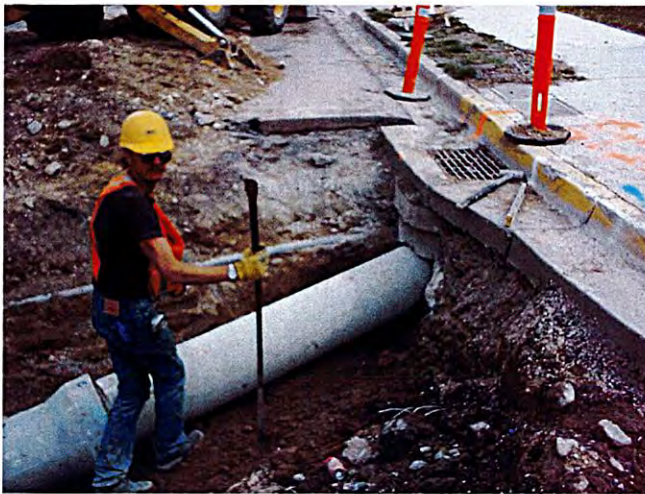
April 8, 2002 Catch basin lateral installation.
