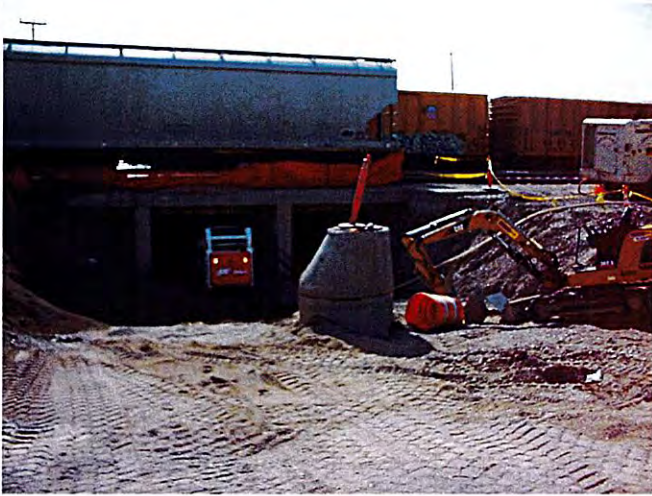
April 1, 2002 Sand backfilling in tunnel on East side.
