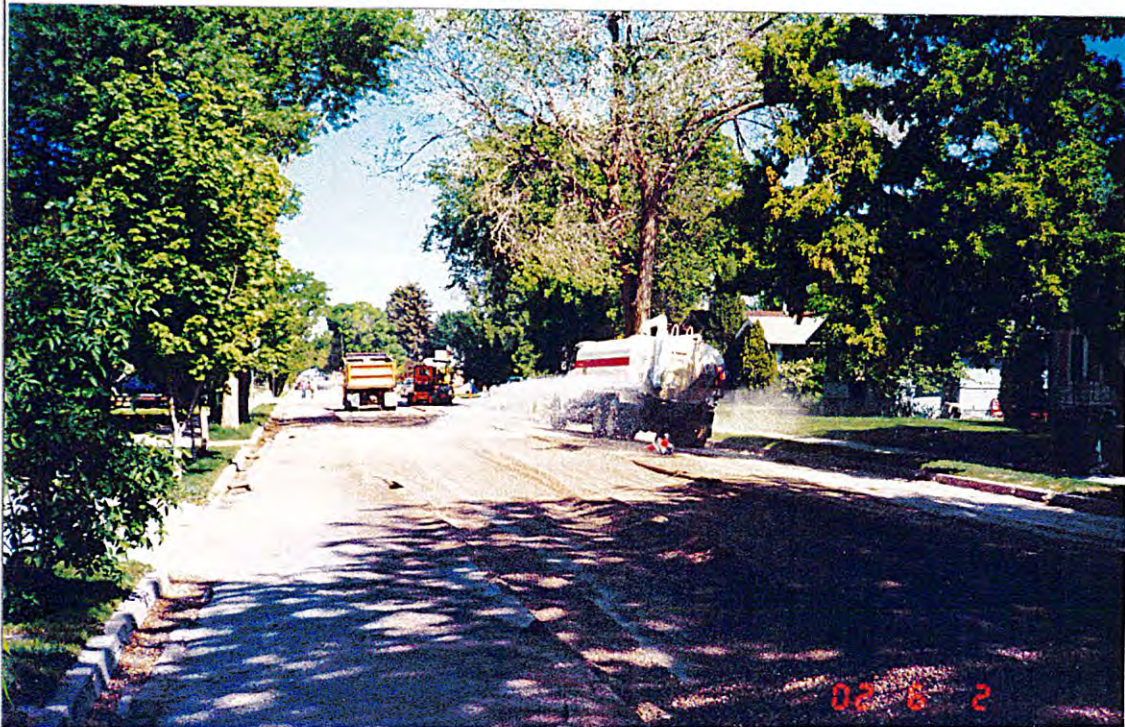
STREET REPAVING PREPARATIONS ON 9 TH AVE.
