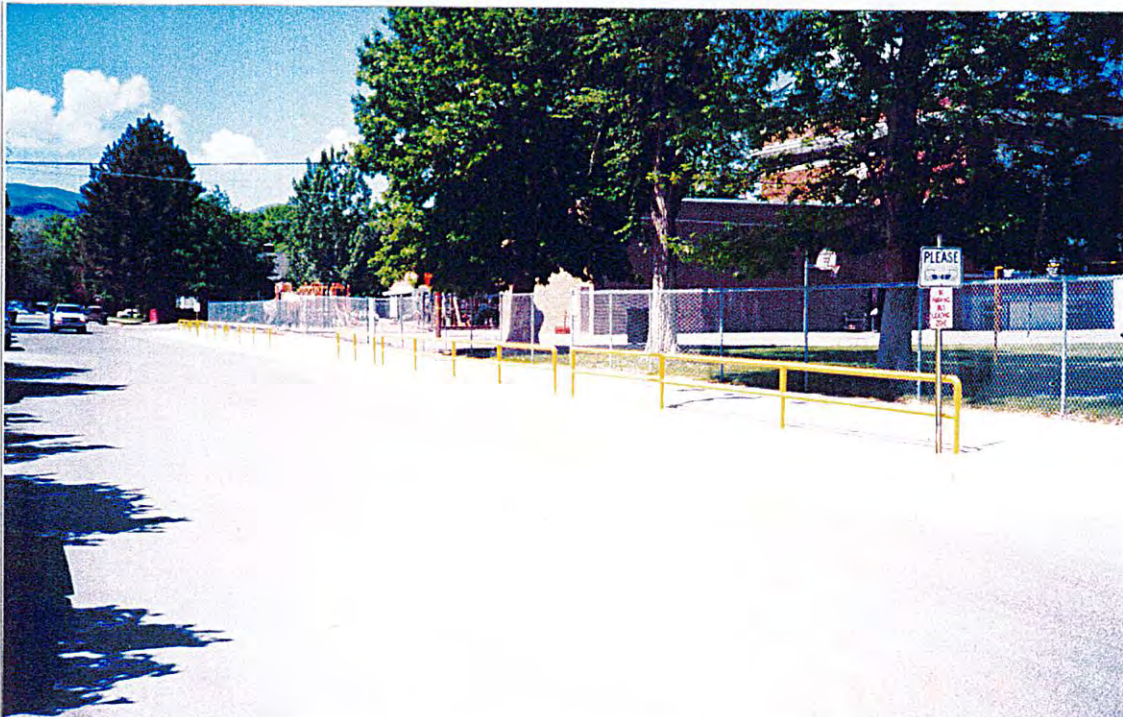
NEW RAILS AND STREET WORK IN FRONT OF WASHINGTON SCHOOL.
