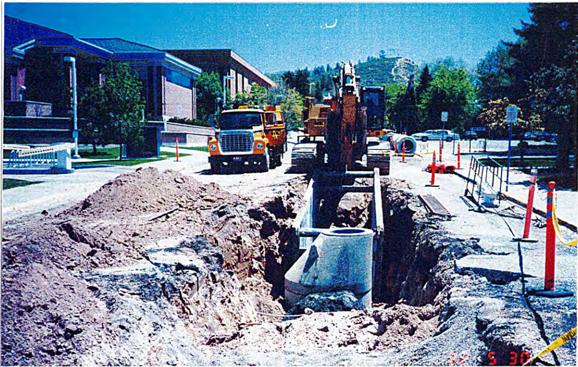
PIPE OPERATIONS ON 9 TH AVE. BY CARTER ST.
