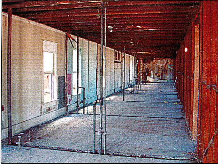
Upper Level Area
