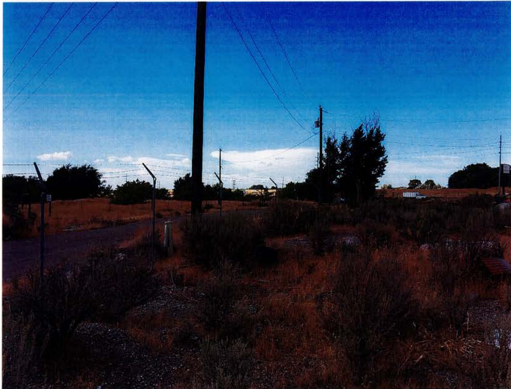
Install safety fence along existing fence line.
