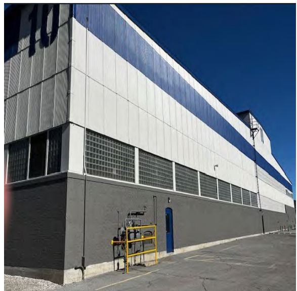
South #10 – Painting – Complete
