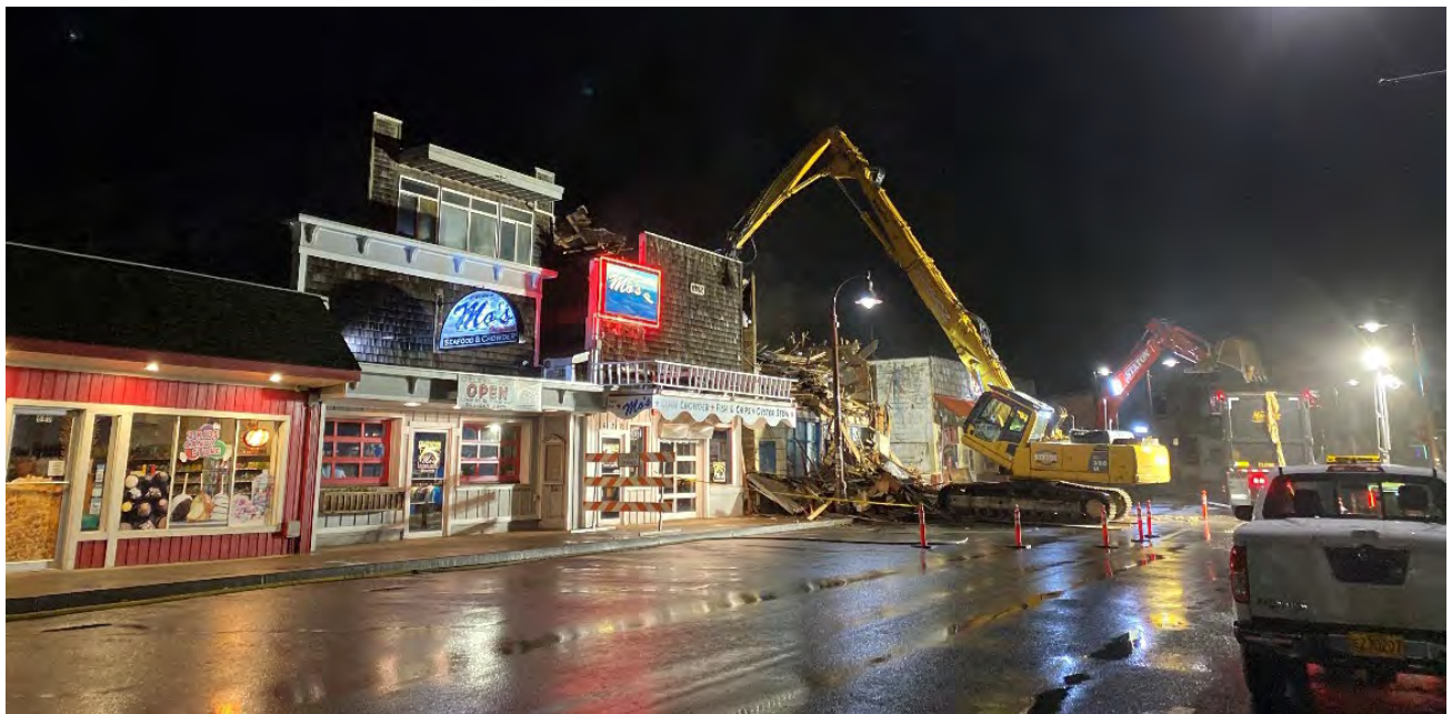
High Reach, 3 Story Building Demo (Night Work), Downtown Newport, Oregon 2024
