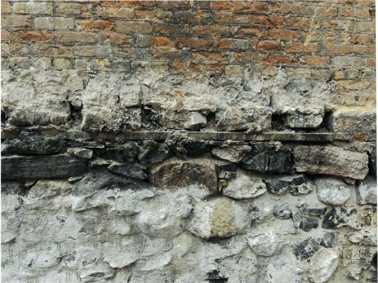
Photo 1 - Existing exposed masonry and embedded wood condition along the Paris Building wall.
