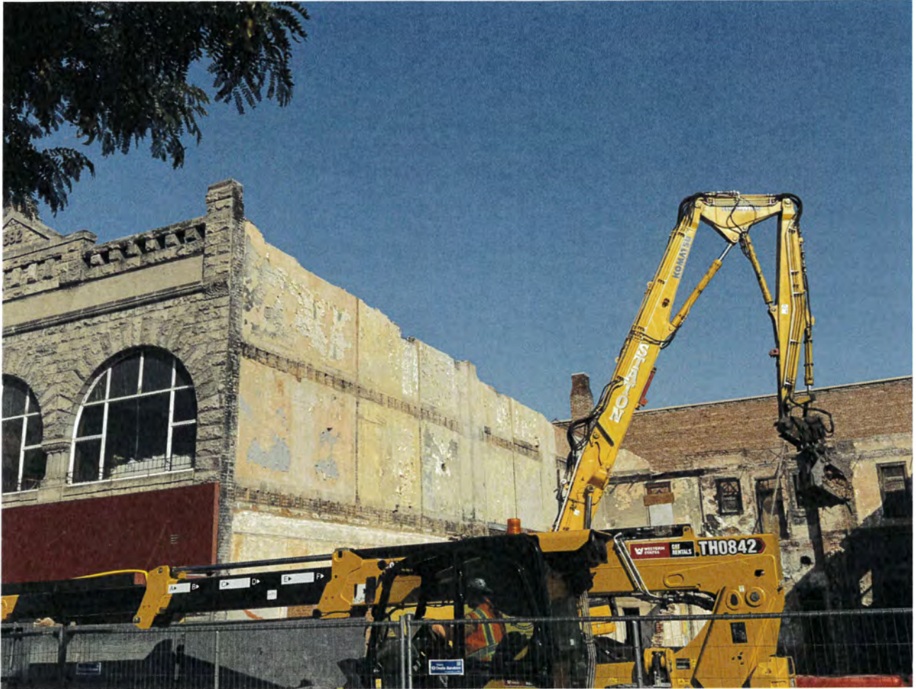
Photo 1 - Paris Building existing condition.
