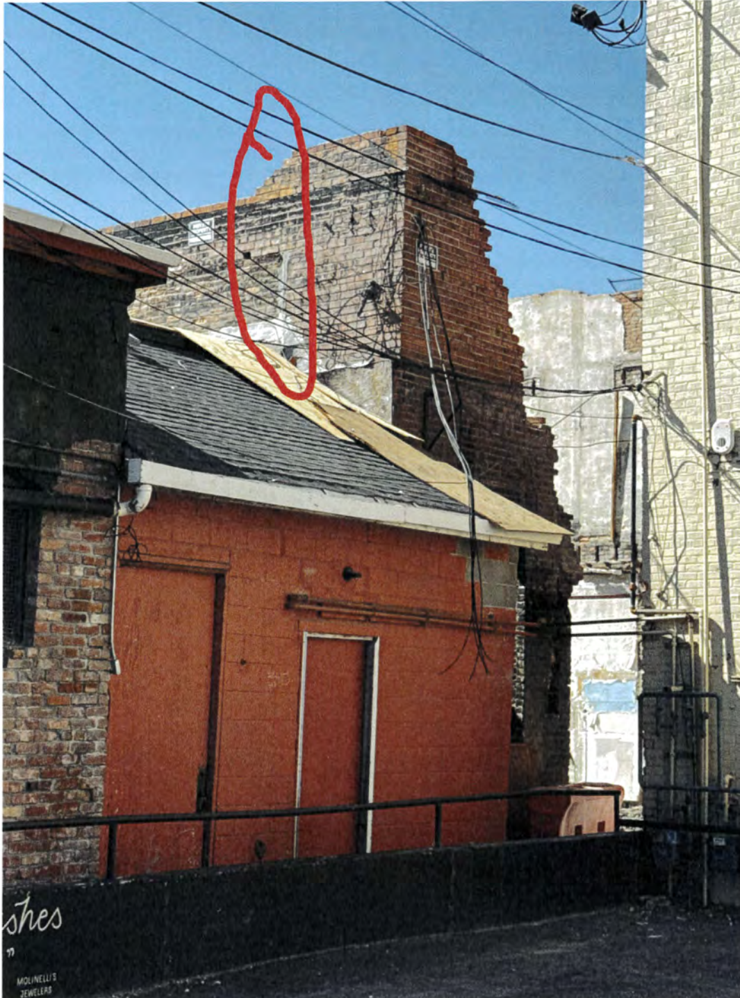
Photo 1 - Exterior view of the remaining perpendicular brick wall; red markup identifies the wall section.
