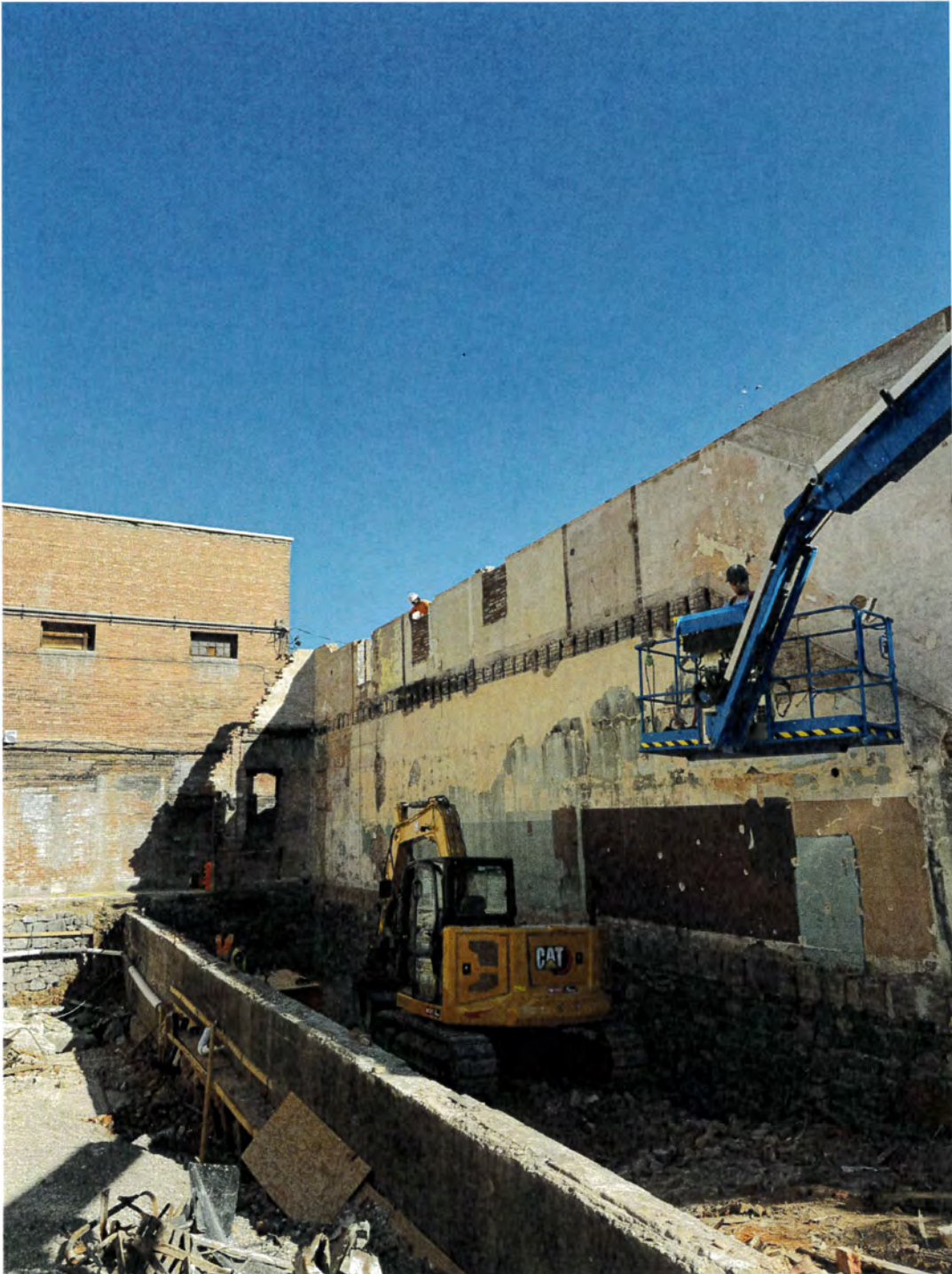
Photo 4 - First National Bar Building window-void infill in progress.
