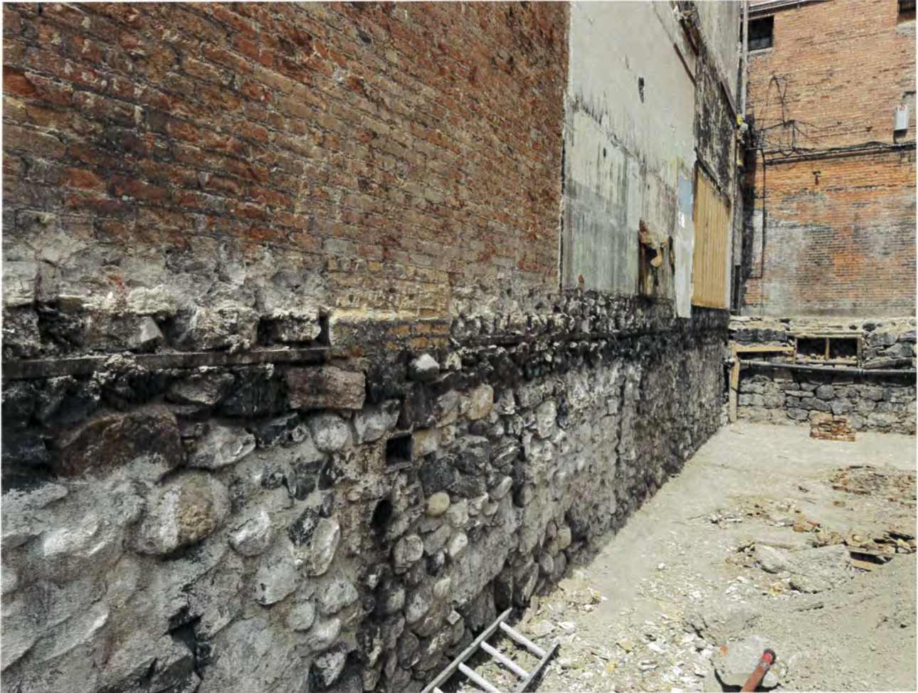
Photo 2 - Overall existing condition along the Paris Building wall.
