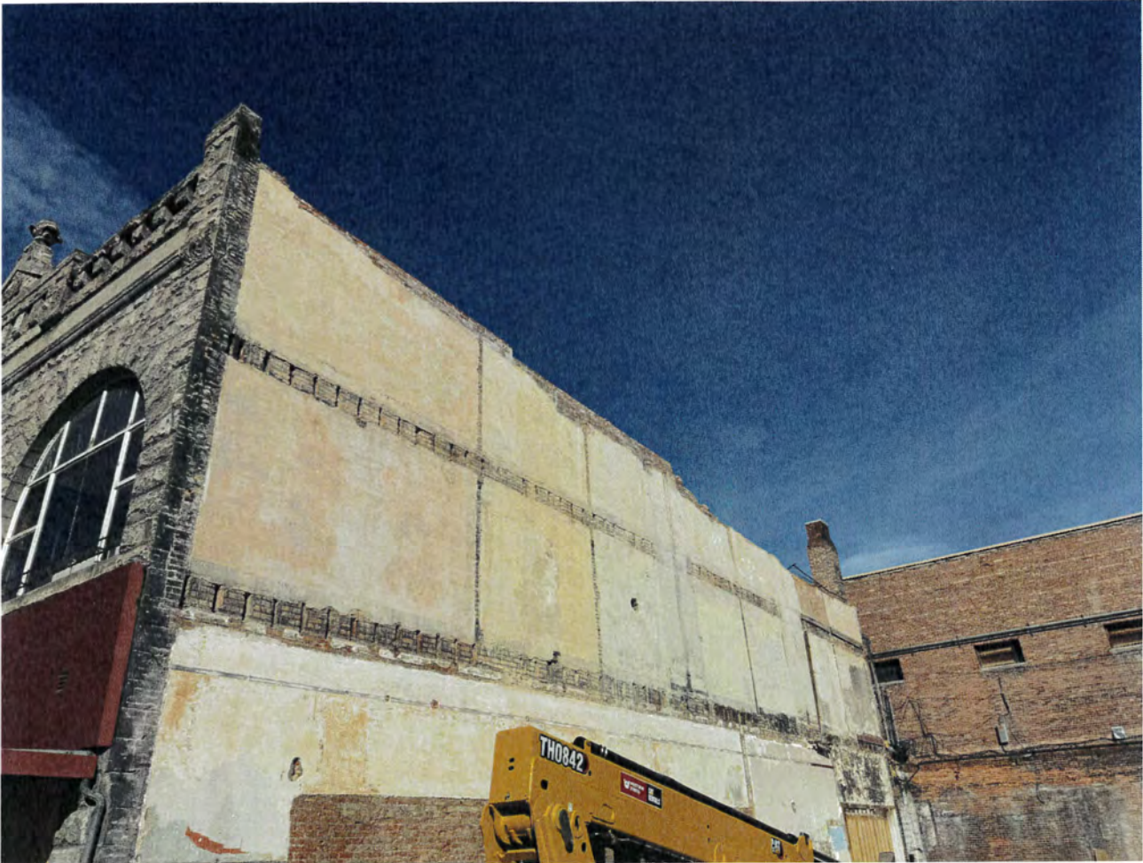
Photo 3 - Paris Building parapet leveling partially completed.
